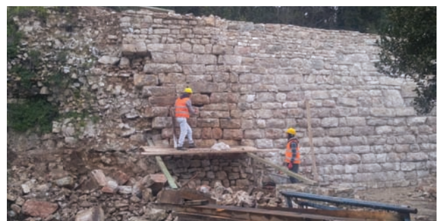
Photo.20-Filling gutters in the southern part of the wall
