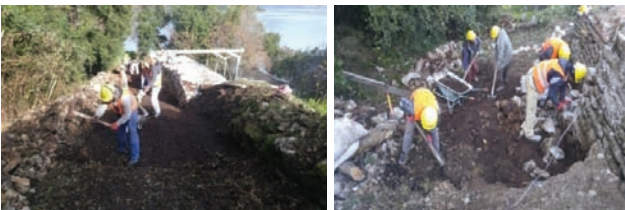
Photo22- The system of demolished stones on the back of the wall
