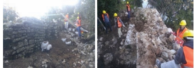
Photo 24- Restoration of the inner wall
