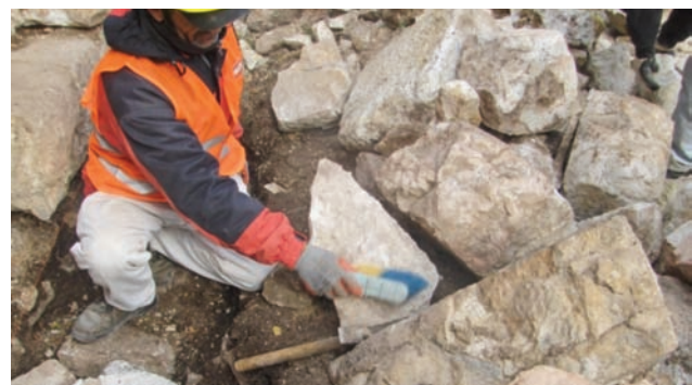
Photo.5 cleaning of blocks from ancient mortar
