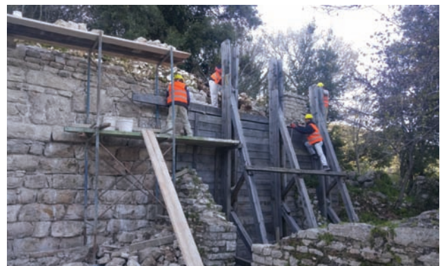
Photo.13-dismantling of the shackles on the north wall
