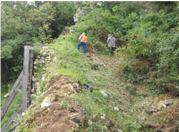
Photo.7-Interior part of the wall before restoration
