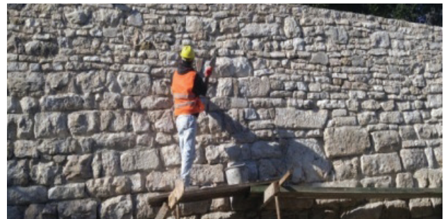
Photo.19-filling gutters in the central part of the wall
