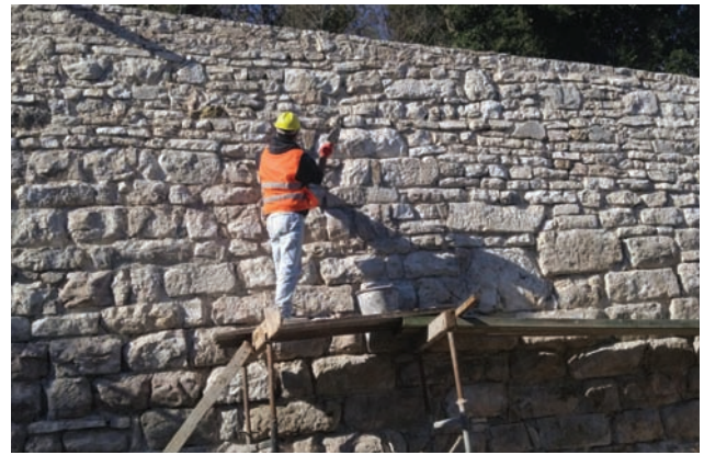
Photo.18-Resettlement of the displaced blocks and their consolidation
