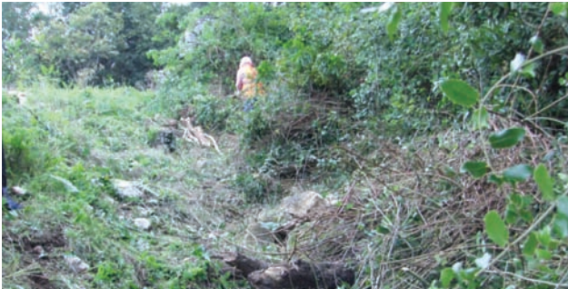
Photo 21- cleaning from the vegetation of the back side of the wall
