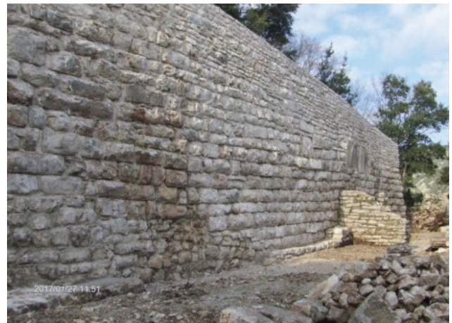
The facade of the wall after restoration
