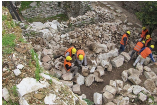
Photo.4 Measuring the blocks for creating rows according to their height and their front page
