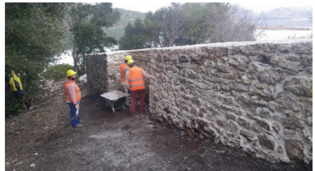
Photo 26-Filling of gutters on the inner wall
