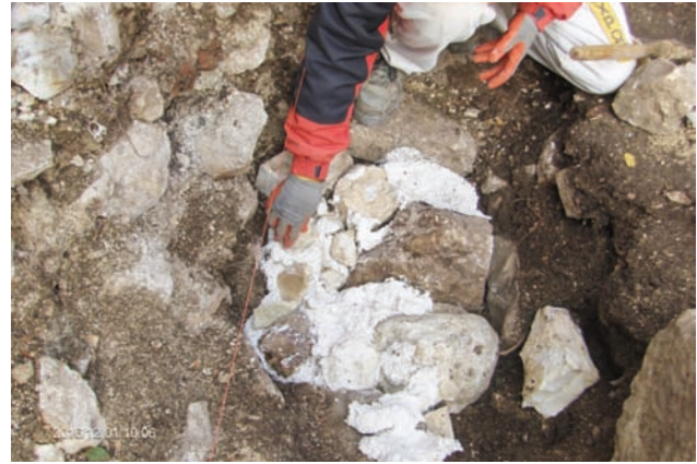
Photo.10-Completing the foundation of the wall
