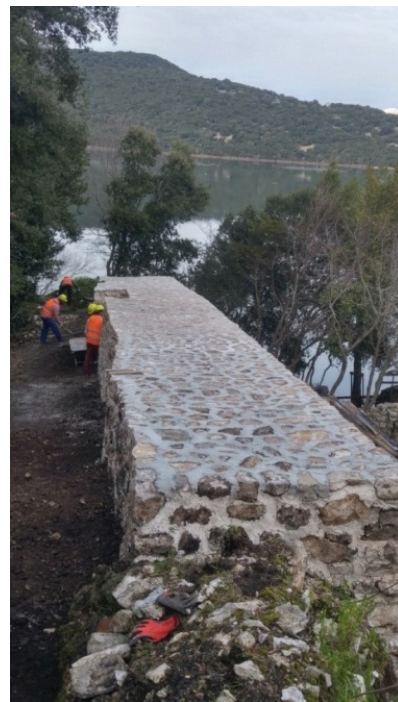
Photo 27- The cap of the wall track
