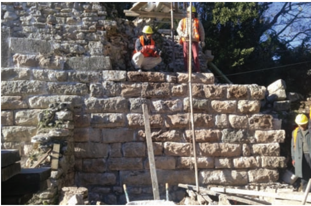
Photo.15-The restoration of the block section on the north wall.
